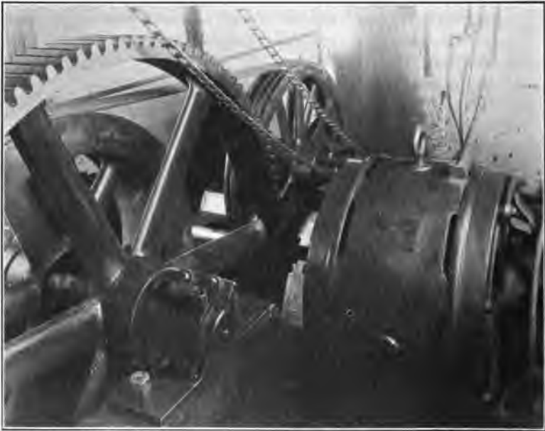
FIGURE 22 TRAMMING PLANT AT THE PENN MINES
